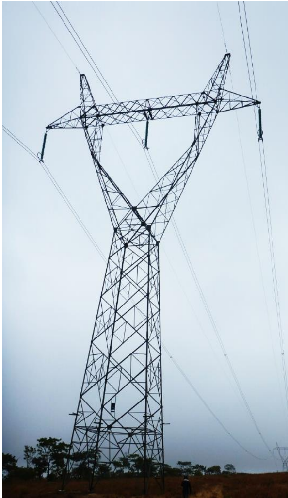
(a) Single Circuit (Not used in the Project)
