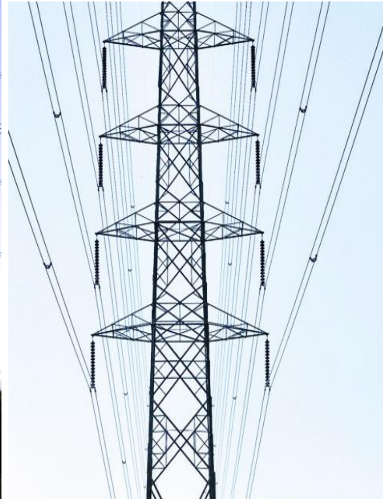
(c) Multi Circuit (used in common corridor Sections)
