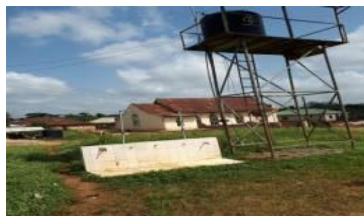
Plate 5.6 Borehole facility in Ekundayo
